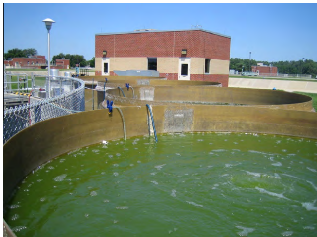
Fig. 1. Algal open pond reactors operated at the Lawrence WWTP, Lawrence, KS. Each of the four 2600-gallon reactors was fed with wastewater effluent from the conventional activated sludge process (influent TN 19.5 \pm 4.5 ; TP 3.21 \pm 0.93 ).
